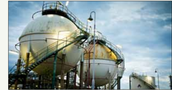
Korea Gas Corporation Substation 21 in Pyeongtaek
