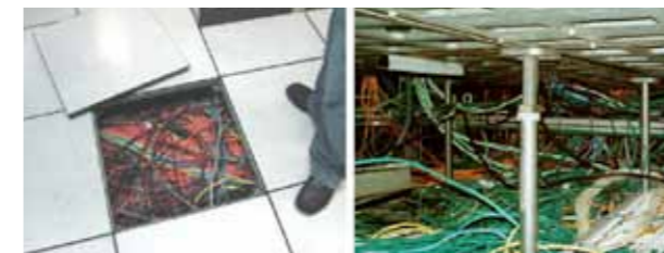
[Figure 3] Cable distribution system in Data Center
