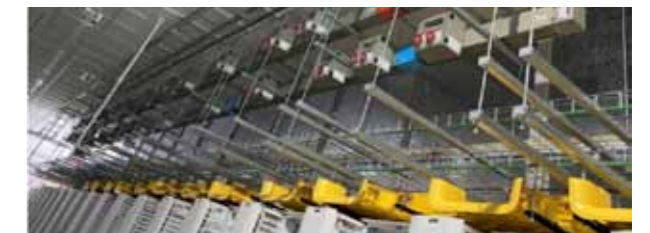
[Figure 4] Busduct distribution system 1
