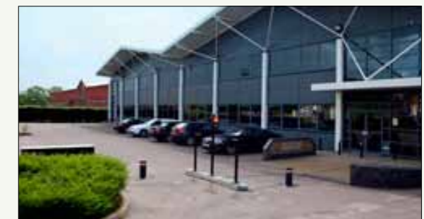
Gyron Data Center Hemel Hempstead, UK, 2012~2013 completed Construction Period : 2012 ~ 2013
