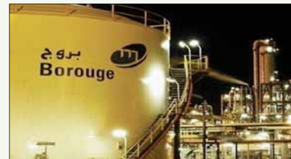
Borough 3 XLPE Abudhabi, UAE, 2012~2013 Will be completed Investor : Borouge Construction Period : 2011 ~ 2013
