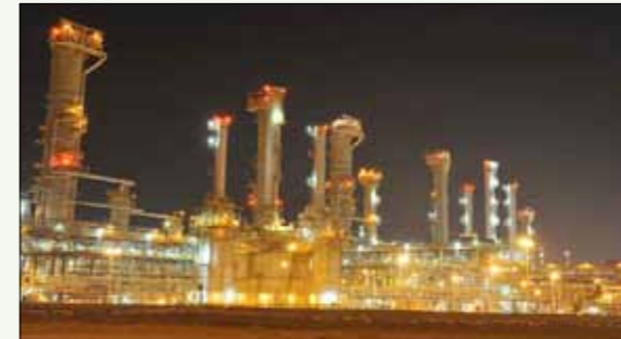
Ruwais Refinery Expansion Abudhabi, UAE, 2012 completed Investor : Takreer Construction Period : 2011 ~ 2013
